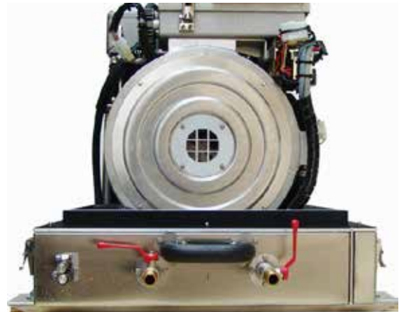
Generator with hot water connection
